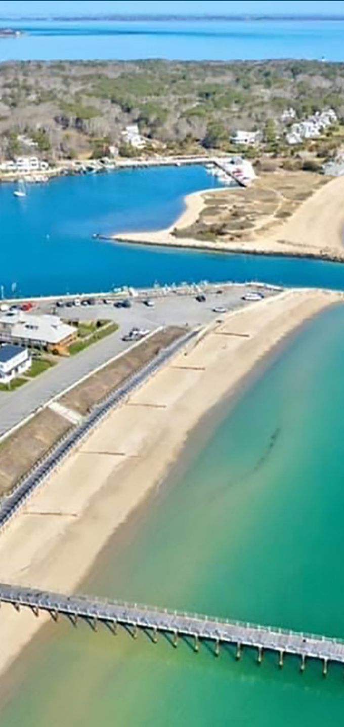
Oak Bluffs Seawall, MA
